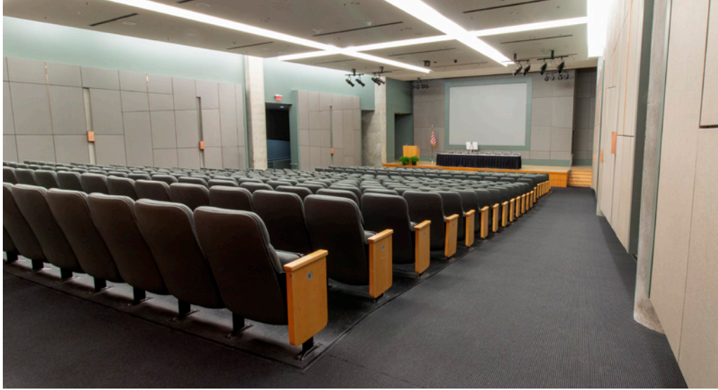
▲ One of the GWCC's three fixed-seat auditoriums that is heated by six dual-fuel VTG boilers.
